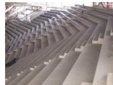
Exposed RCC structure
